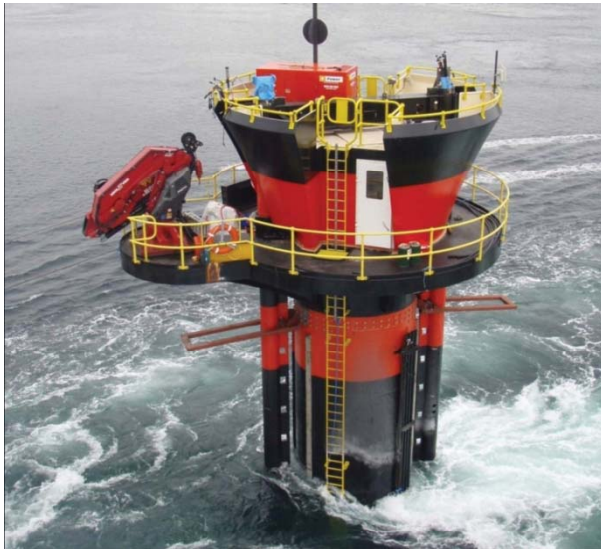
The 1.2 MW SeaGen tidal flow generator in Northern Ireland's Strangford Lough.
